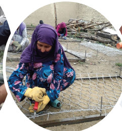
Gabion weaving flood mitigation, Afghanistan
